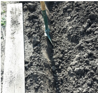
4. Dig a trench.
