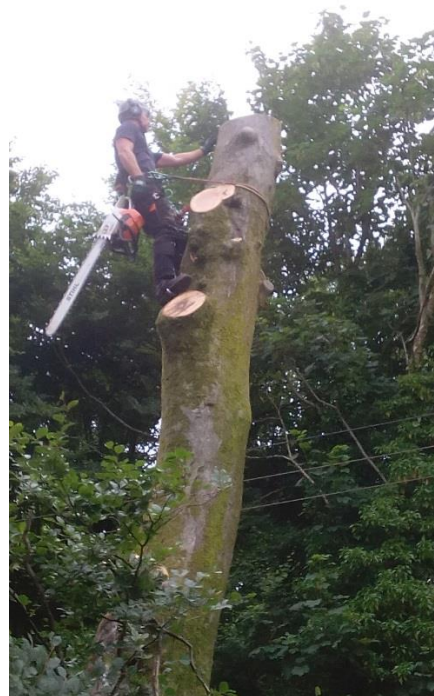
Matt Evans – utility site dismantle job
