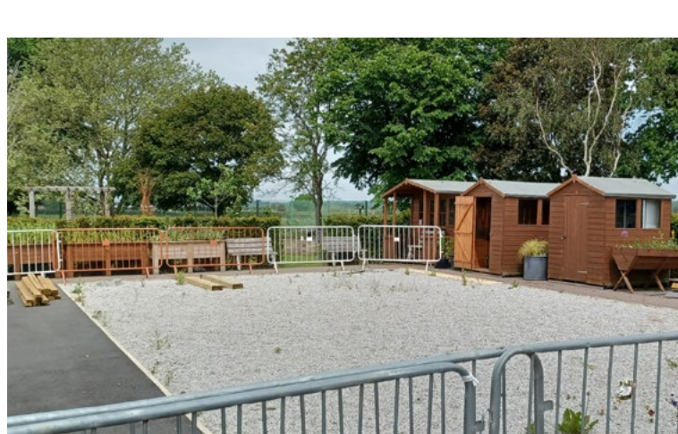
Preparing to start building on the Village Green.
